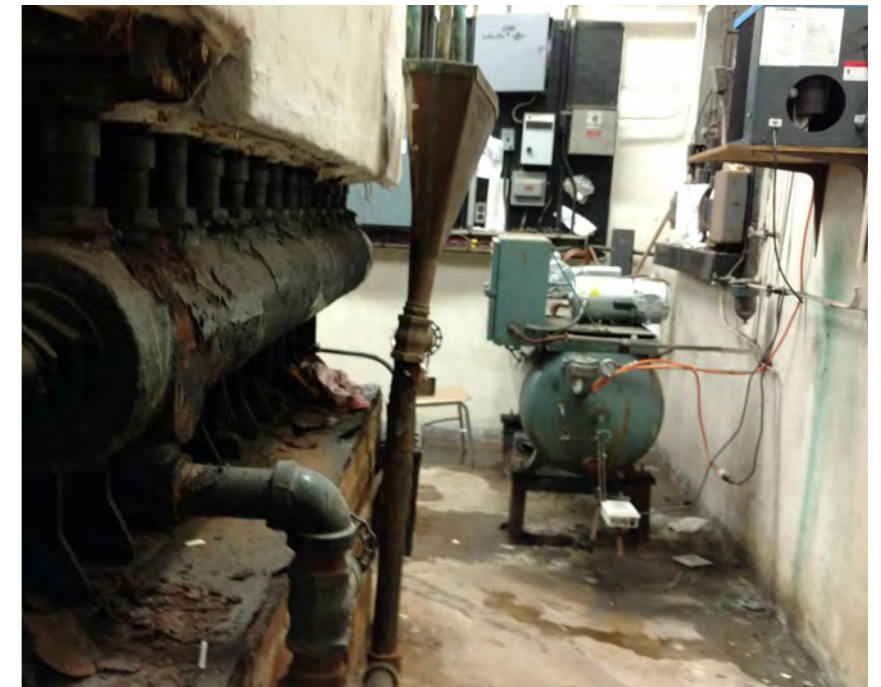
Corrosion at boilers
