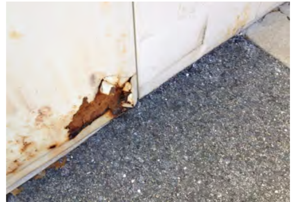
Rusting Panels at the 1974 Addition
