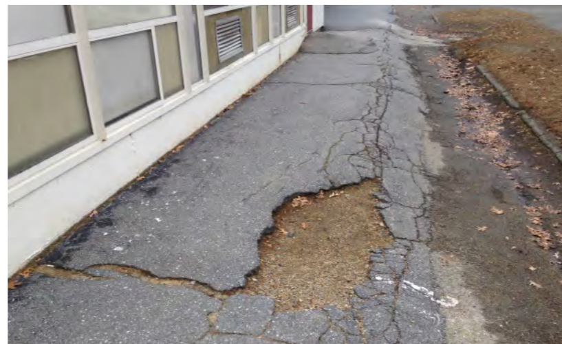
Deteriorating asphalt
